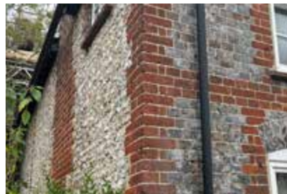
Brick bonding and mix of brick exterior finishes
