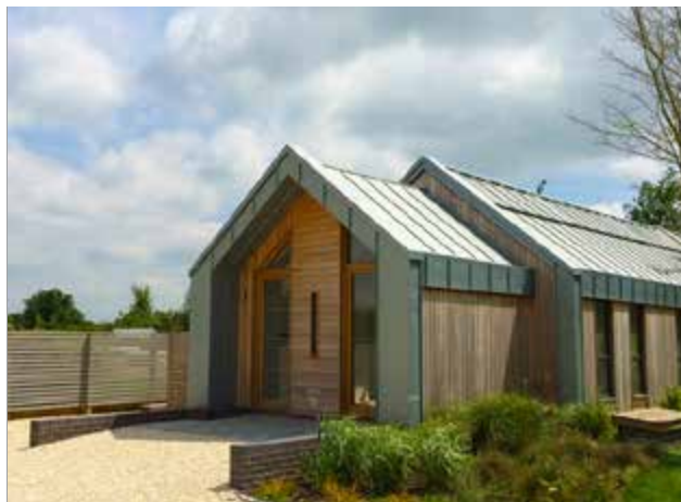
F.72 Office unit with appropriate materiality for a rural location. Elsewhere in the UK. Source: https://find-an-architect.architecture.com
