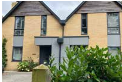
Light brick and timber frame exterior finish
