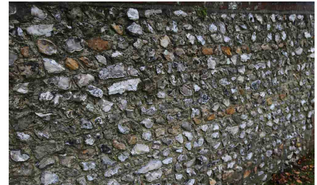
Figure 34: Red brick and facing flint wall.
