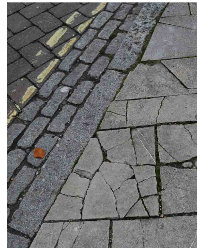
Figure 41: Paving damage
