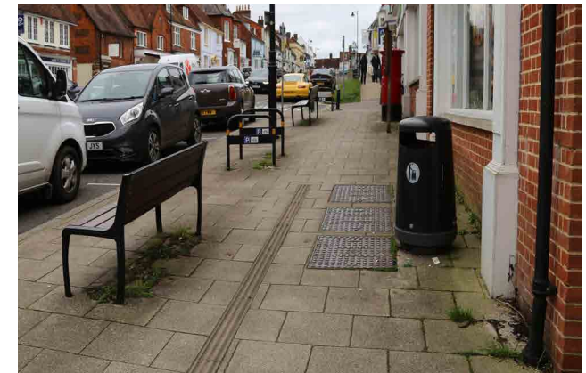
Figure 46: Weed growth around street furniture.
