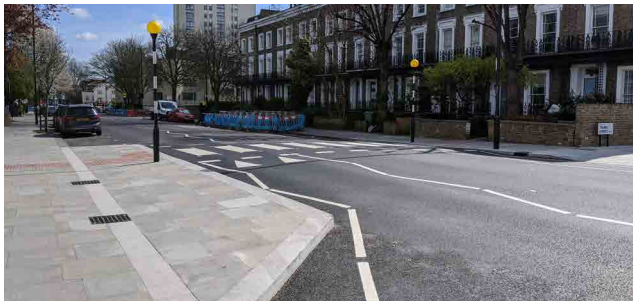
Figure 89: New build-out to provide crossing. Co-located with PRow and public convenience.
