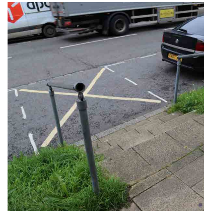
Figure 32: Level change from pavement to street.
