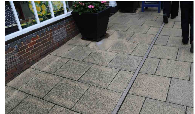
Figure 35: Purbeck stone paving.
