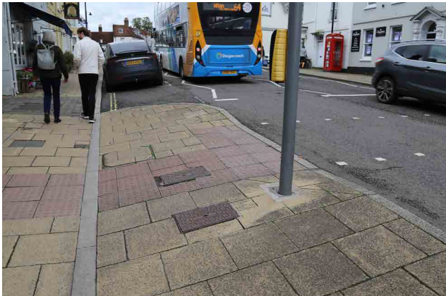
Figure 37: Image emphasises the camber and level change, with huge implications on surface water management.
